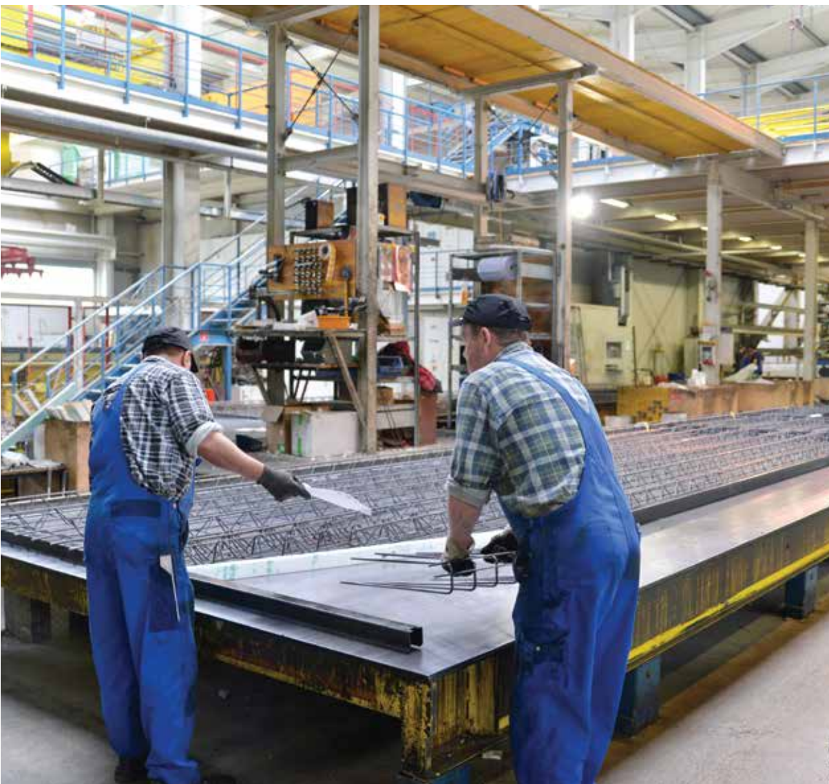
Precast Facility Spread across 73,000 sq ft
