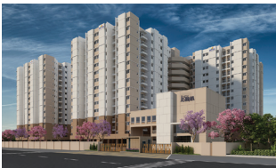
ASHRAYA Bengaluru-Mysuru Expressway Bidadi
